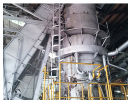
Waste heat recovery
