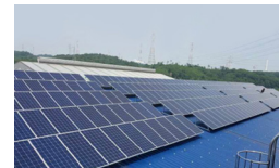
Comas Solar photovoltaic power plant (286kW)
