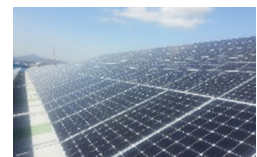
JHG Power photovoltaic power plant (372kW)
